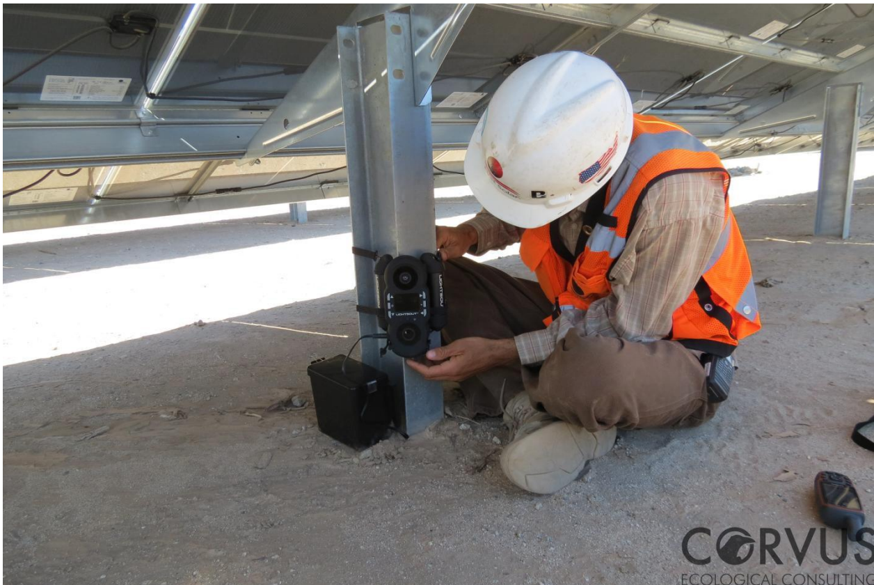
Figure 3. Installation of a game camera within a solar array.
