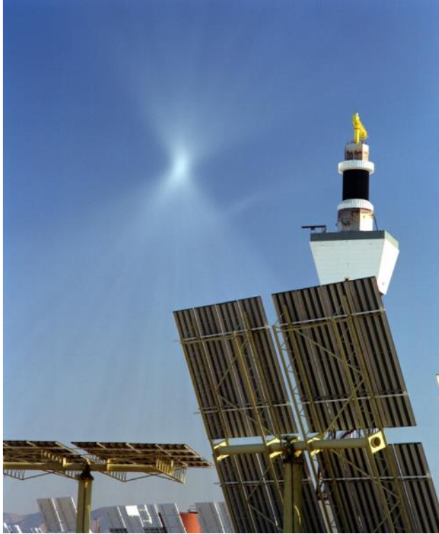
FIGURE 3 Glow of Scattering Sunlight from Heliostat Beams Converging on a Point Near the Tower During Operation of the Solar Two Demonstration Plant in 1996 (Photo credit: NREL)
