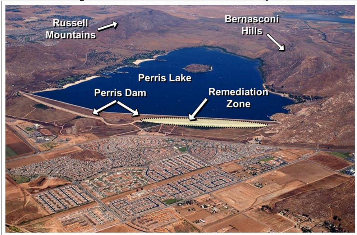
Figure 12-1: Perris Dam Construction Project 65
